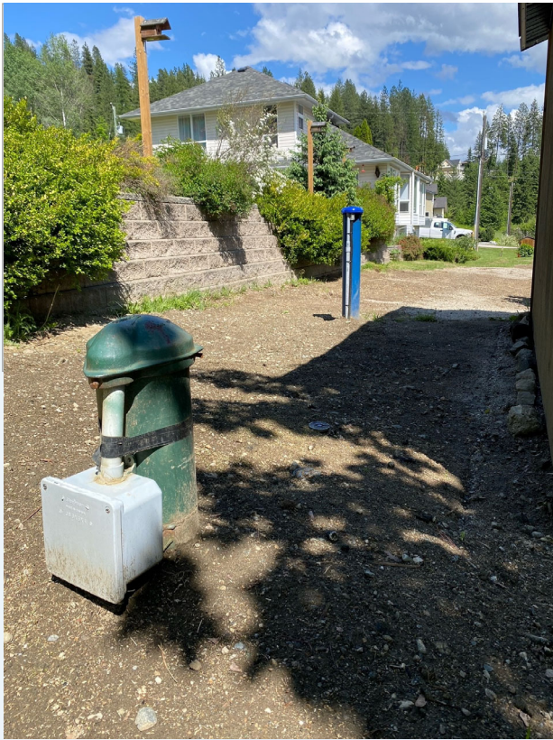
New well site remediation
