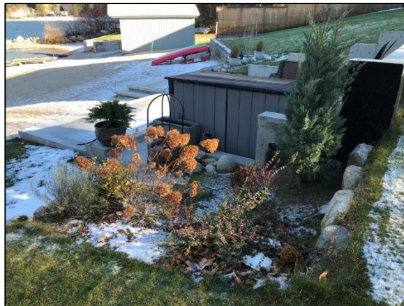
Photo 12. View of vegetation on the west side of the concrete foundation. Nov. 17, 2022.
