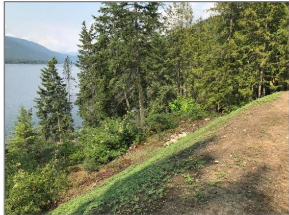
Photo 8. View of upper limits of riparian area and embankment descending from housing development.
