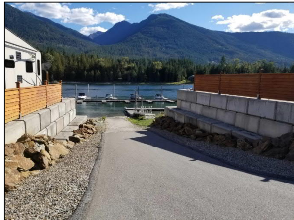
Photo 5. View of boat ramp and tie back lock block retaining walls looking south, Sept 16, 2021.
