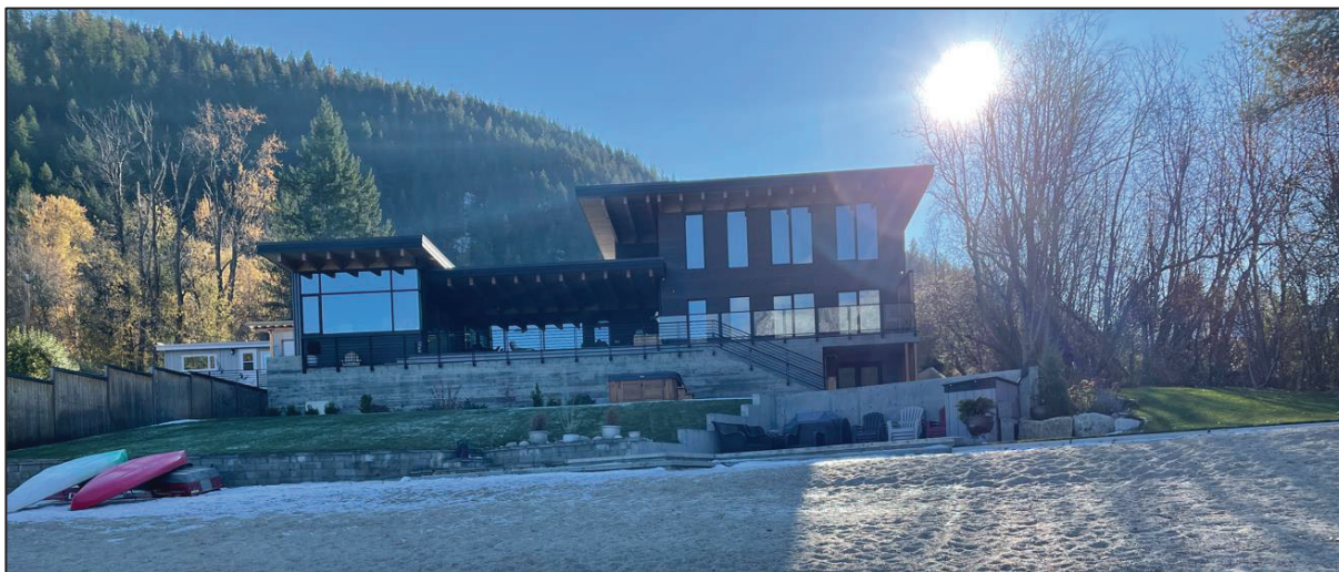
Photo 4. View of property post-development. Nov 17, 2022.
