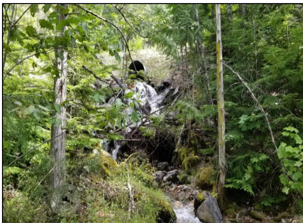
Photo 11. Upstream view of Wilmot Creek towards highway culvert crossing.
