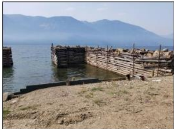
Photo 10. View of breakwater structure south of property, Sep 8, 2021.
