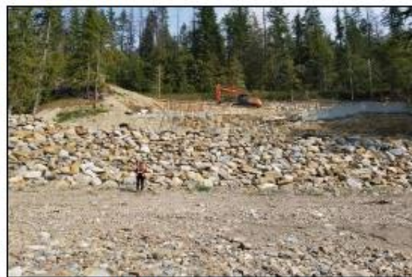
Photo 4. View of re-grading within riparian setback, Sep 8, 2021.
