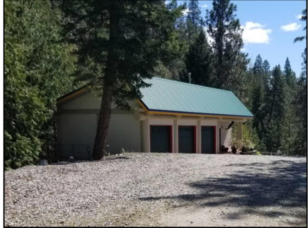
Photo 6. View of cleared parking area and garage next to residence.
