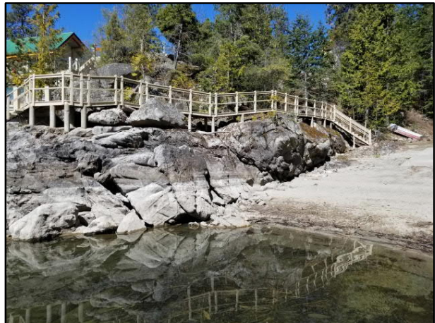
Photo 10. View of wooden walkway and stairs.
