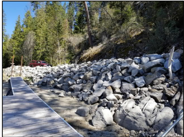
Photo 8. View of raised area armoured with riprap at boat launch area.
