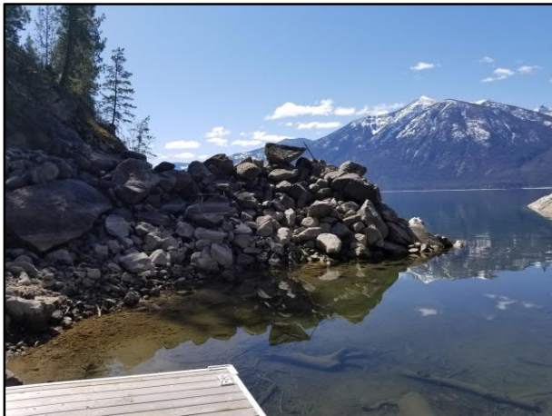
Photo 9. View of rock groin.
