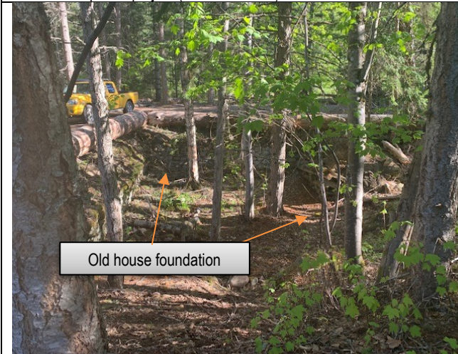
Photo 3: Trees growing in old house foundation (east view)
