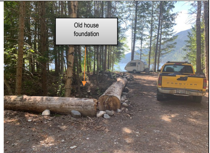
Photo 4: Logs placed as protection around the old house foundation (southwest view)
