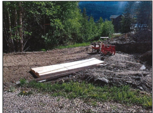
Photo 6. Excavation for cabin 1 next to creek
