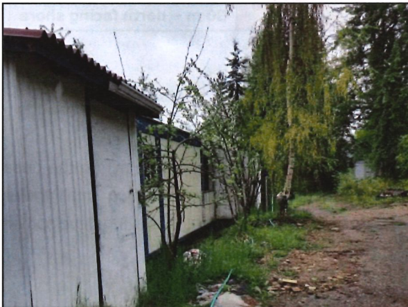
Photo 5. West side of existing mobile home where 1.22 m wide addition will run.
