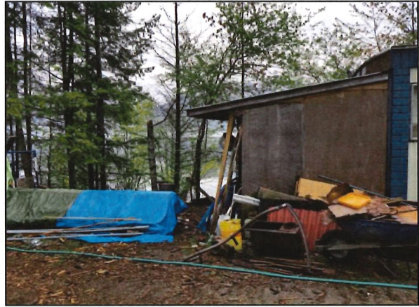
Photo 4. View east to proposed workshop footprint. Note the trees in the left corner which will be removed.
