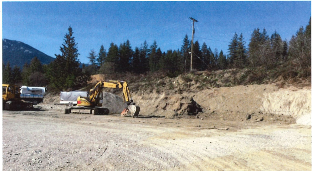
Proposed site of the building. Photo taken facing west.
