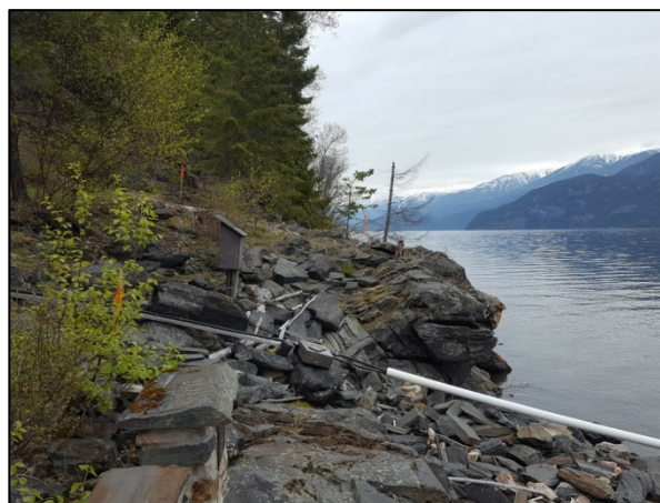
Photo 5. View of rocky shoreline looking north from in front of proposed meeting room.
