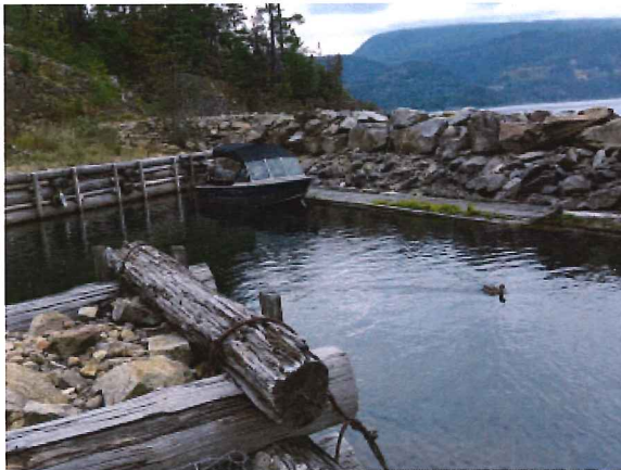
Photo 8. North-west view of breakwater structure, log cribbing and dock.
