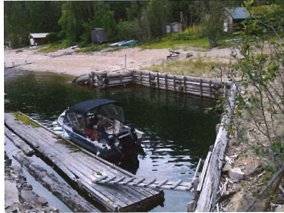
Photo 9. South-east view of dock and log cribbing along shoreline.
