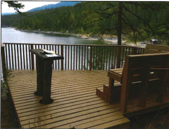
Photo 3. View of sundeck located within trees at north-west corner of Lot 2.
