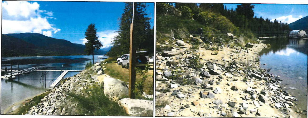
Figures 4 and 5. Existing rip-rap on Lot C (left) and the foreshore of Lot B with water levels close to the natural boundary (right).
