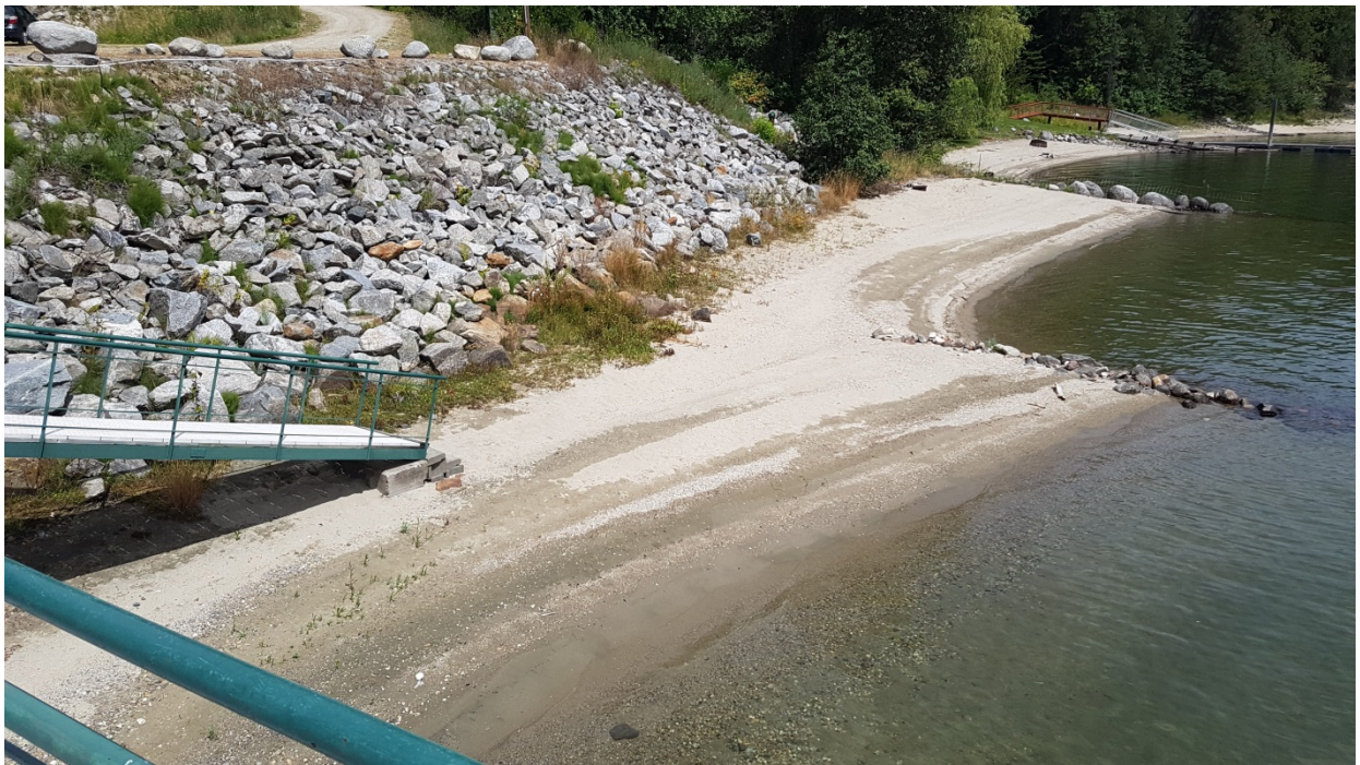
Figure 7: View of Foreshore Area of 6744 Highway 3A
