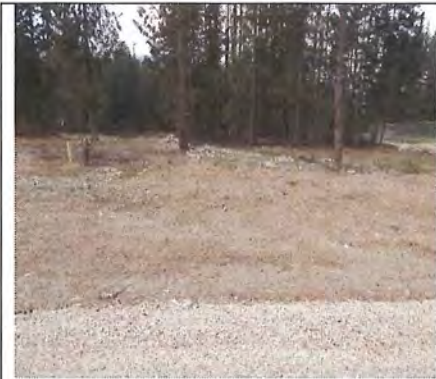
PHOTO 1: East end of Lot 1 (west view)
