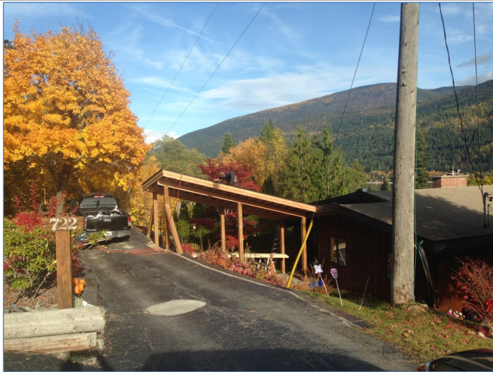
Figure 3: Covered walkway build within Stromme Lane right-of-way
