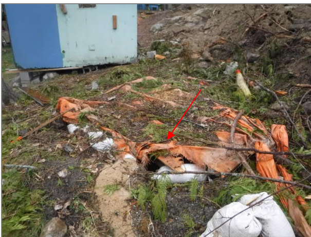
Photo 5. View of Hall Spring (abandoned) southwest of pumphouse
