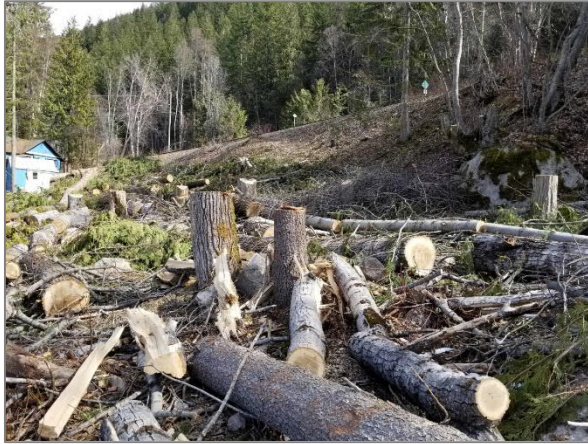
Photo 3. View of cleared trees looking east.
