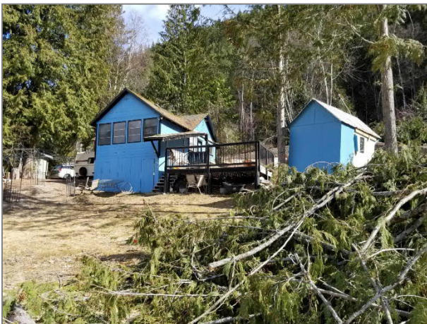
Photo 7. View of one-bedroom cabin, deck and pumphouse.
