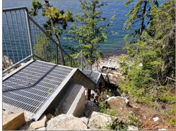
Photo 12. View of partially constructed metal grate stairway and deck (July 26, 2023).
