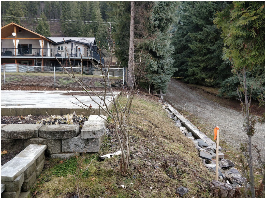
Figure 7 – View looking east that shows the 1.5 metre distance from the existing concrete slab to the property line.
