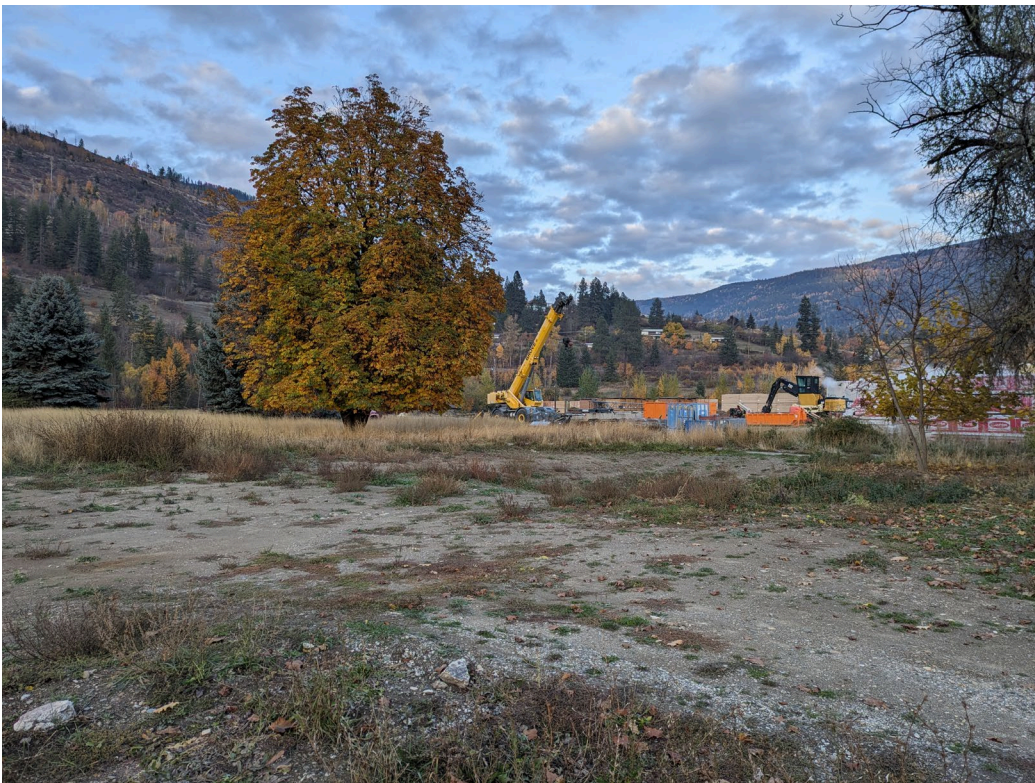
Figure 6 – Location of the original dwelling that was destroyed by fire.
