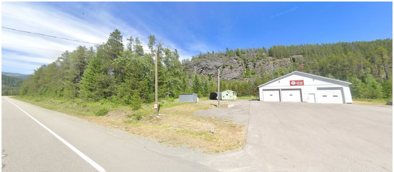
Figure 4: View of Subject Property from Neighbouring Fire Hall
