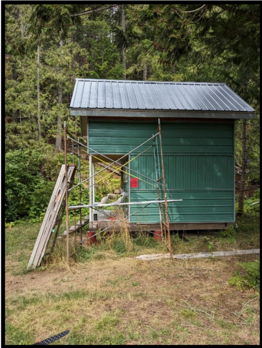
Photo 1. Aug 24, 2023 - Photo of SWO placed
