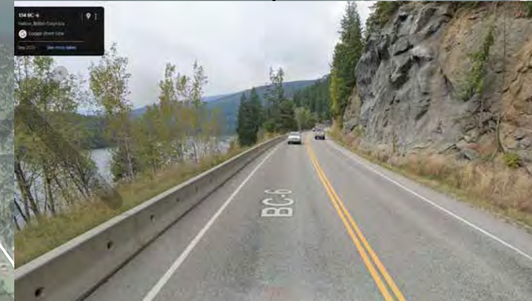
Constrained HWY ROW - Building on the slope north of the HWY will be very difficult and expensive. Using Fortis transmission line ROW may be more feasible.
