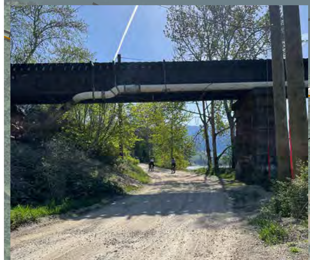
Road crossing beneath train bridge
