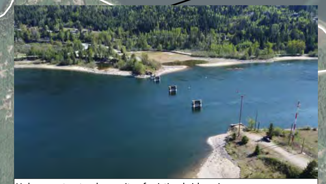
Unknown structural capacity of existing bridge piers
