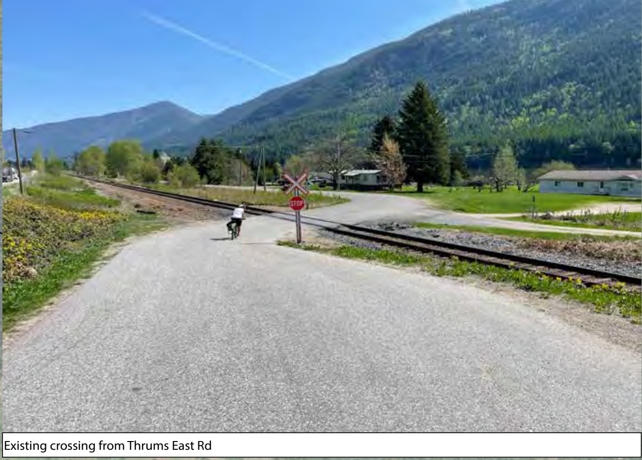
Existing crossing from Thrums East Rd
