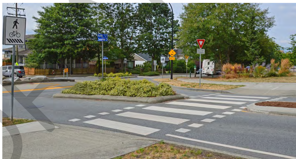
Figure 14: Combined Cross-Ride and Crosswalk on the Spirit Trail in North Vancouver
