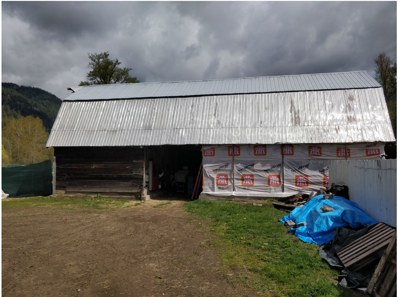
Figure 1 - View north facing the existing agricultural building that shows the breezeway between the two portions of the building. The left side of the building will be used for horses and the right side of the building will be converted to a dwelling.
