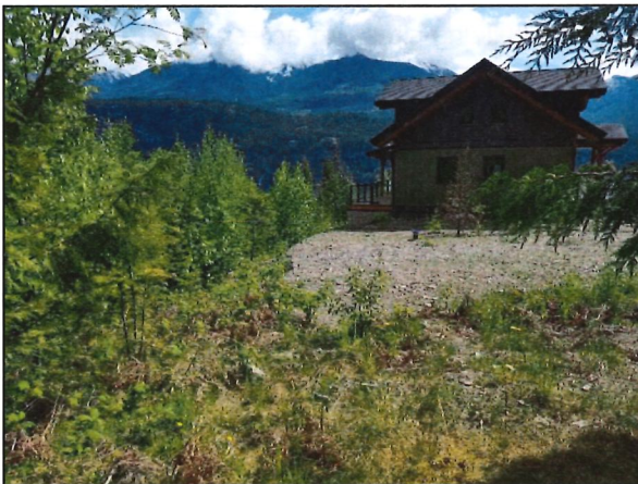
Photo 5. Recently completed cabin 3.
