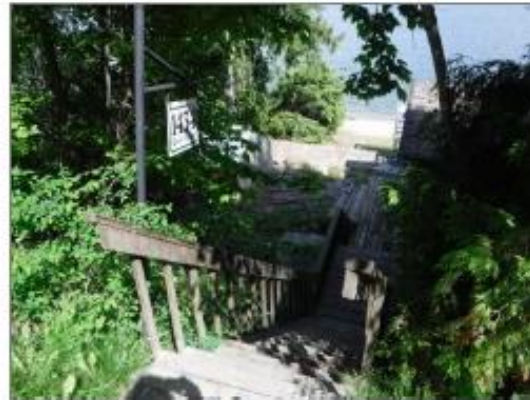
Photo 2. View of highway embankment staircase.
