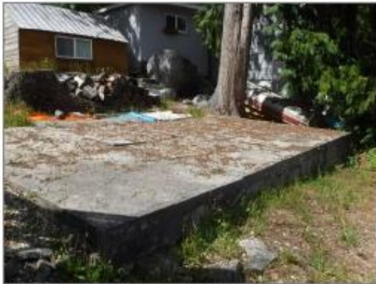
Photo 3. View of concrete slab patio.
