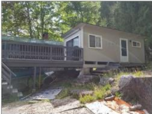
Photo 1. View of existing cabin and raised deck.
