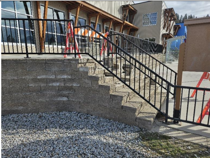
Gap Between Stairs "B" and Concrete wall
