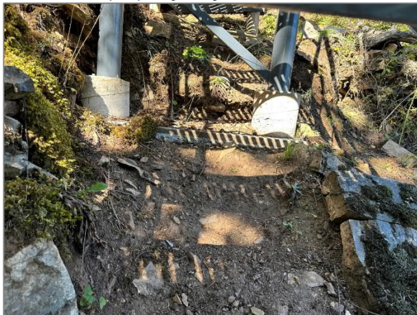
Photo 9. Disturbed soil under stairway
