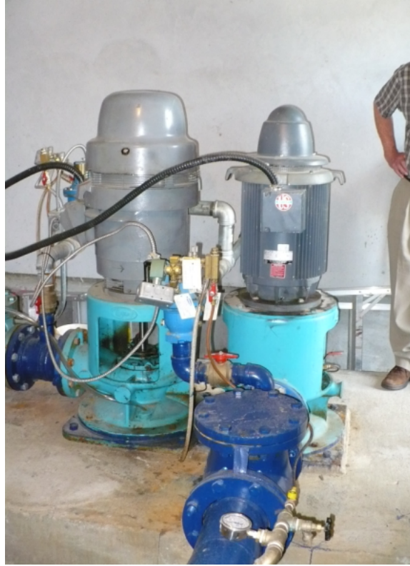
Balfour Pumphouse, August 13, 2009
