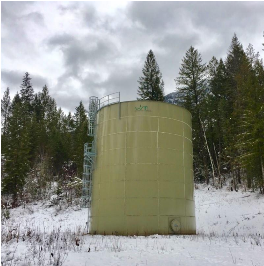
Figure 1: Finished Storage Reservoir
