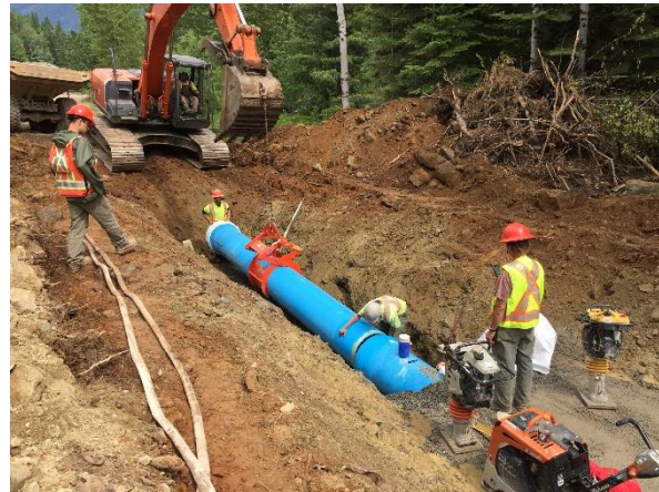
Arrow Main Line Replacement
