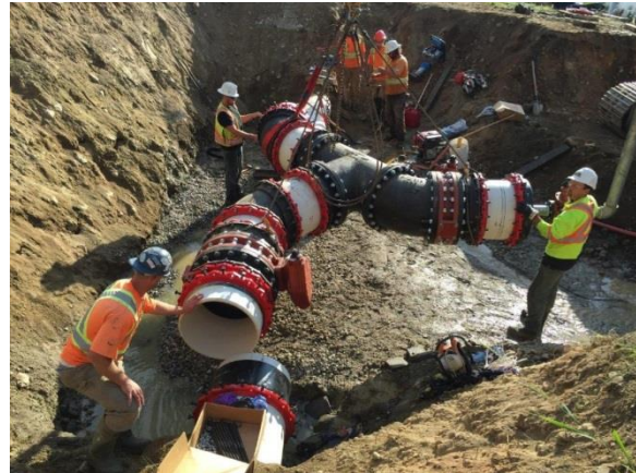
Arrow Mainline Replacement
