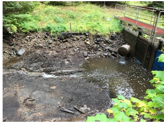
Ymir Water Intake
