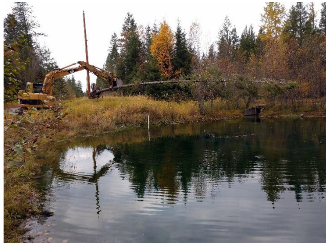
Wetland Construction at Old Lister Intake
