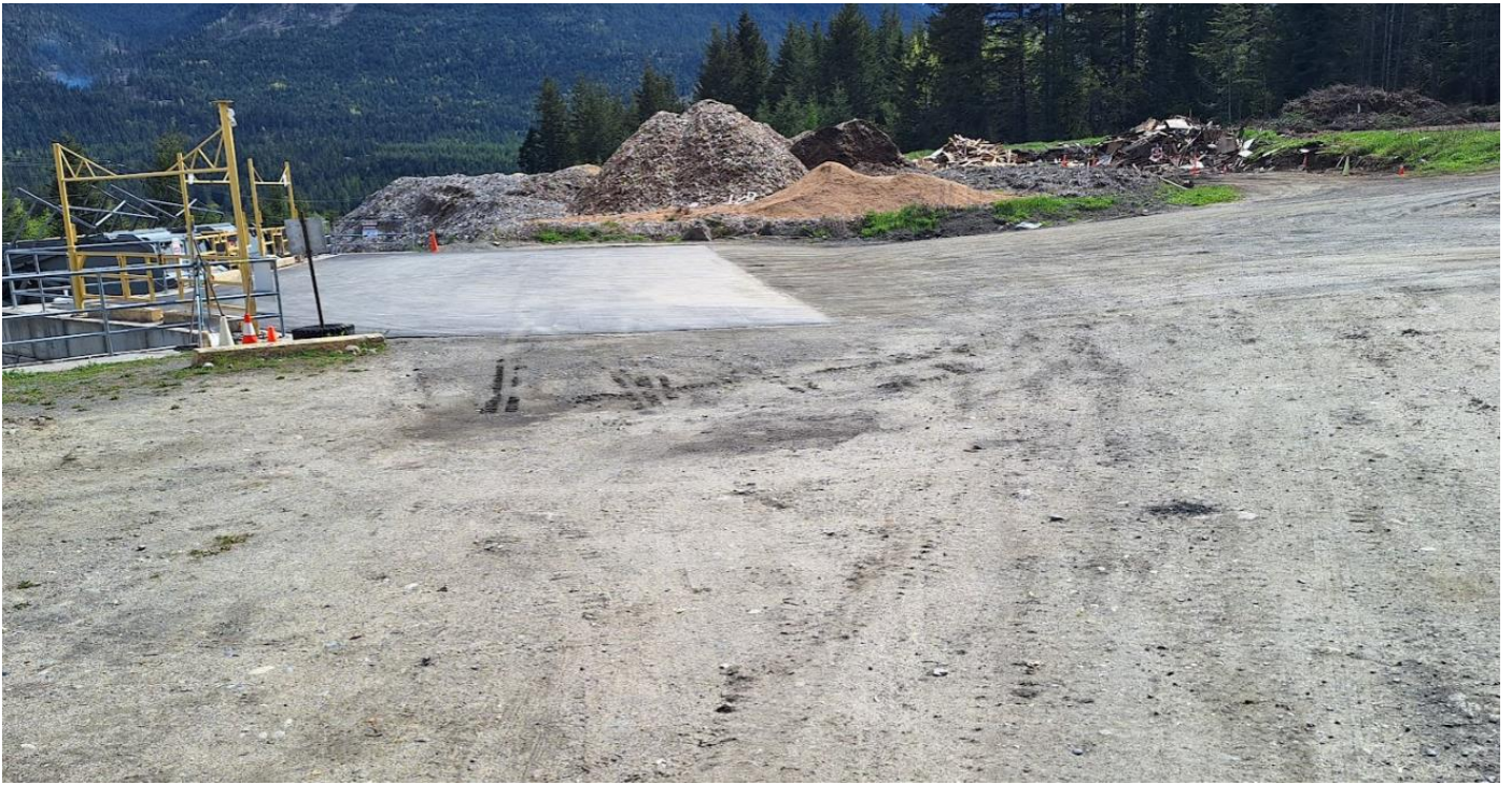
Site regraded following paving.
