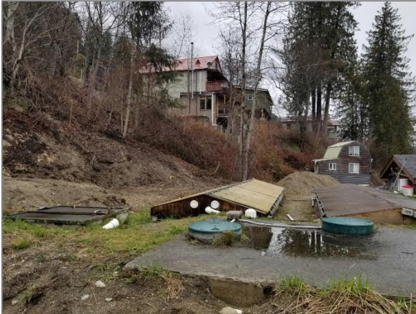
Photo 3. View of WWTP and expansion area looking north.
