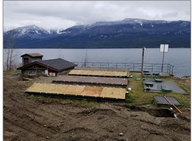
Photo 4. View of WWTP looking east.
