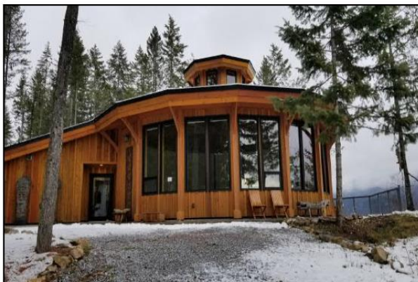
Photo 1. View of Roundhouse located on 5278 and 5308 Amundsen Road.
