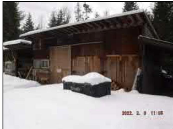
Photo 12. Front view of equipment garage.
