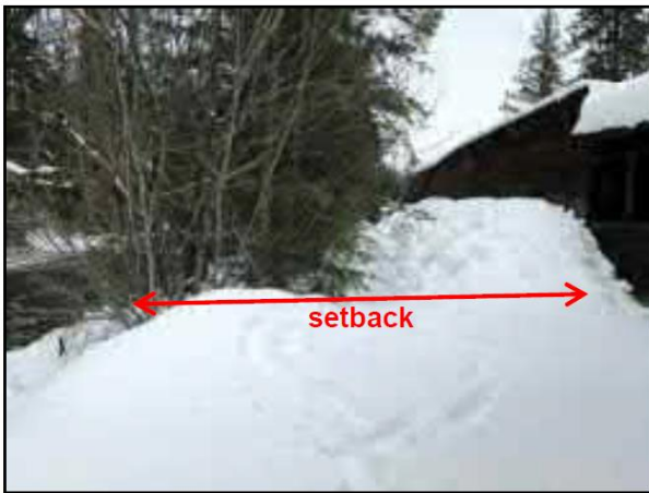
Photo 13. Rear view of equipment garage and setback from Erie Creek, looking north (upstream).
