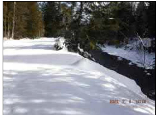
Photo 6. View of dyke or old road along the southern property boundary and Erie Creek looking east (downstream).
