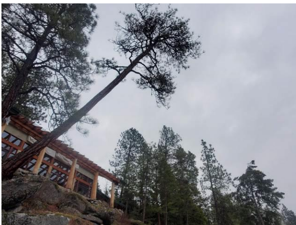
Photo 5. Leaning ponderosa pine view southeast leaning over SPEA.
