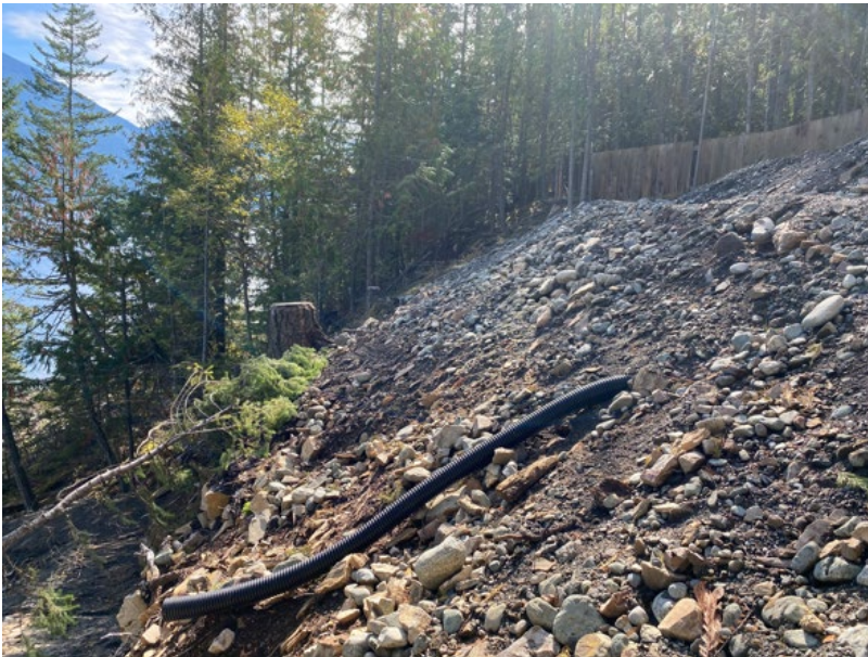
Figure 13. Slope of Zone 6 to be improved with CWD anchoring, slope texturing, and possible soil bioengineering using willow.
