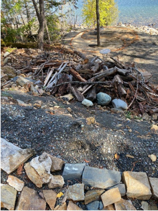
Figure 12. CWD from Zone 3 to be situated on Zone 6 hill prior to topsoil placement.
