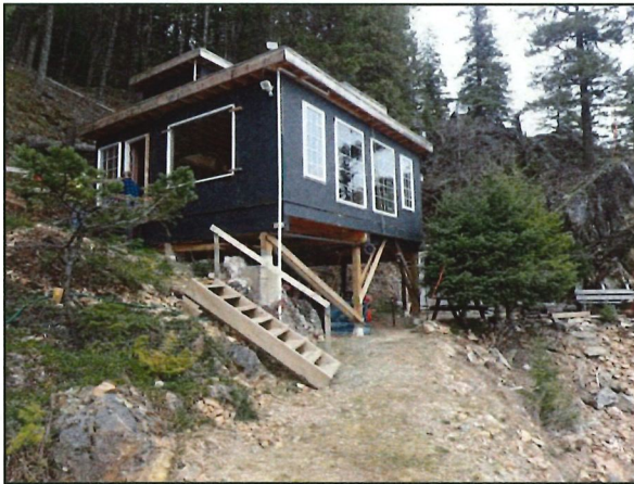
Photo 3. Existing cabin constructed on bench within the 30 m WDP and 15 m SPEA.
