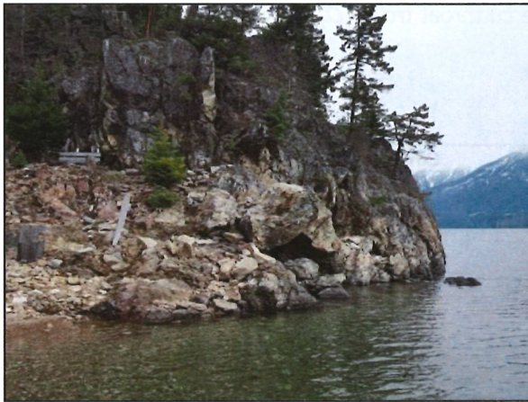
Photo 11. Shoreline composed of rocky cliffs and boulders on the north edge of the property.
