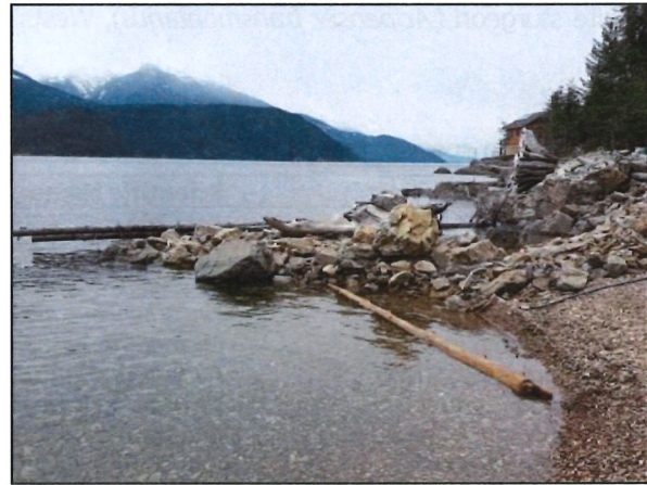
Photo 12. South view of rock groyne in front of subject property.
