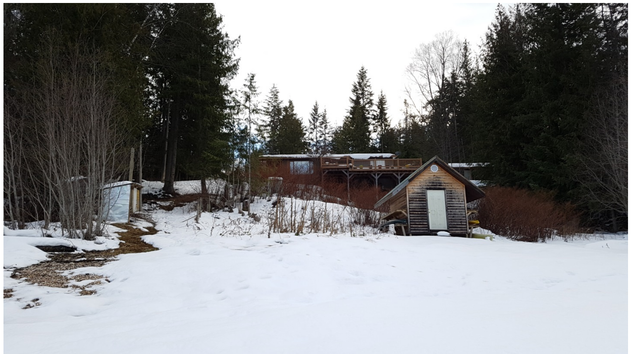
Figure 4: View South of Small Shed and Single Family Dwelling at 16828 Fraser Subdivision Road
