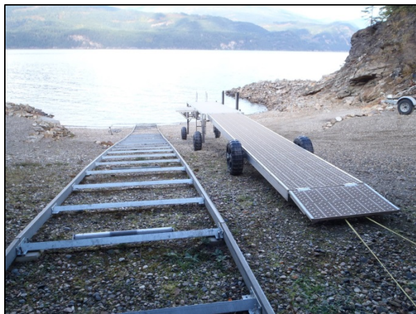
Photo 18. Example of marine rails.
