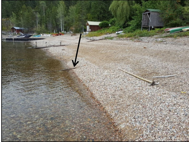
Photo 7. Water intake line for Lot 2.
