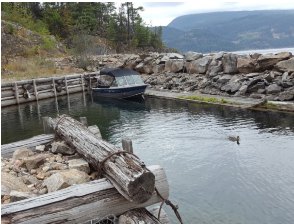
Photo 8. North-west view of breakwater structure, log cribbing and dock.
