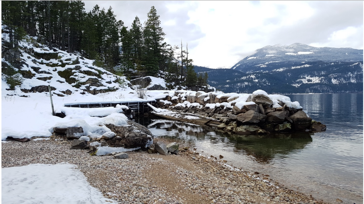
Figure 5: View of Existing Moorage Facility in the Foreshore Fronting 16828 Fraser Subdivision Road
