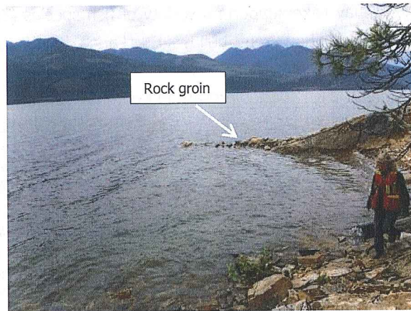
Photo 14. Rock groin location on the north side of boat access.
