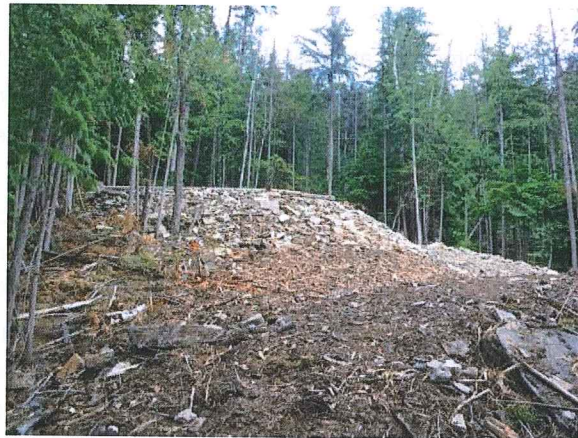
Photo 6. Clearing and re-grading completed on Lot 3.
