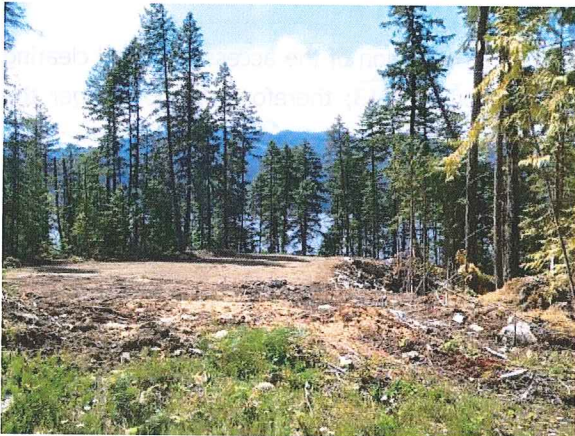
Photo 5. Clearing and regrading completed on Lot 2.
