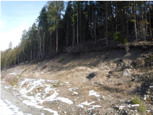
Photo 6. View of exposed cut bank above septic field.
