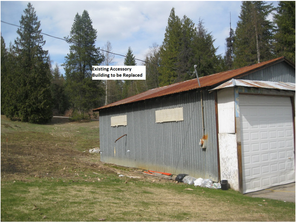
Figure 3: Existing Garage to be replaced by Accessory Building with Secondary Suite Above
