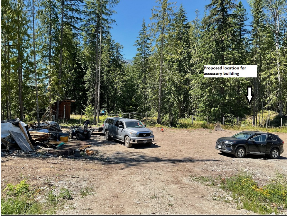
Figure 3: Area cleared and prepared for building
