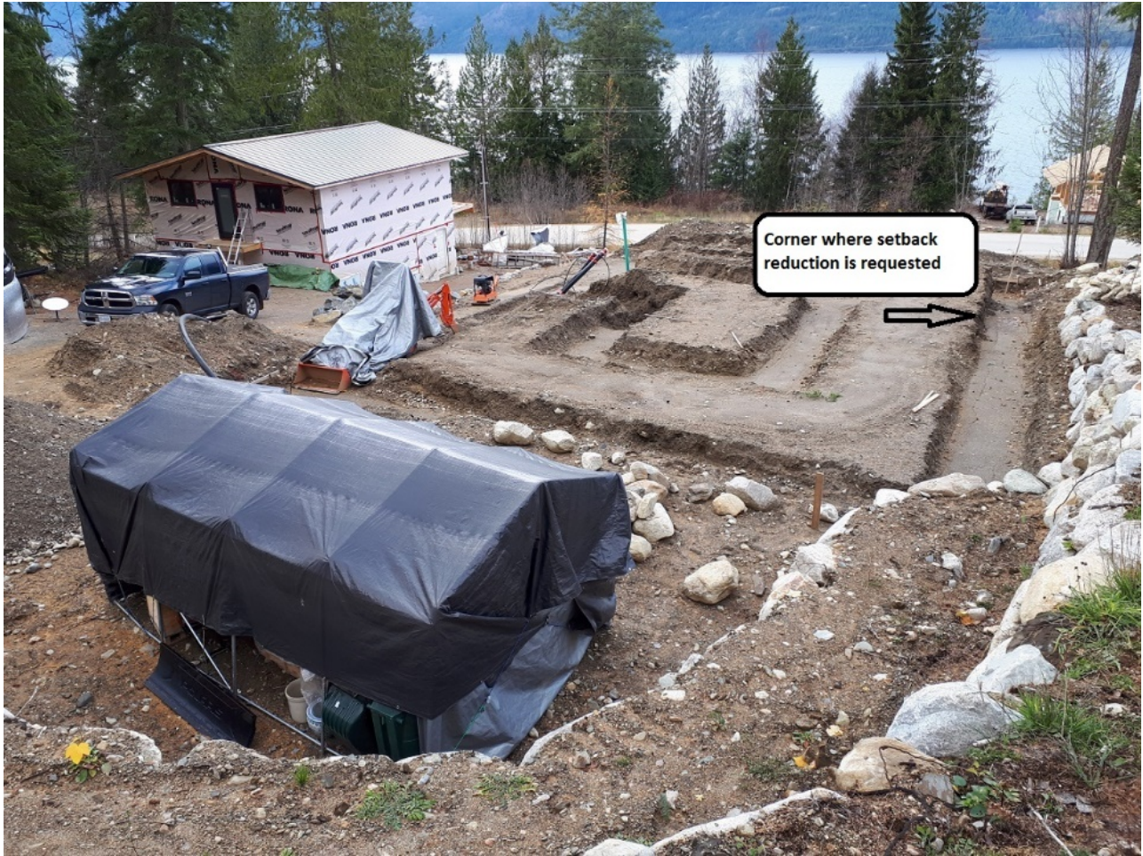
Figure 4: Building Site during Snow Free Conditions
