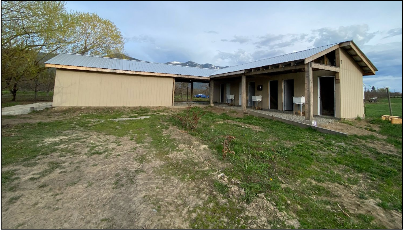
Figure 3: Photo of Existing Structure
