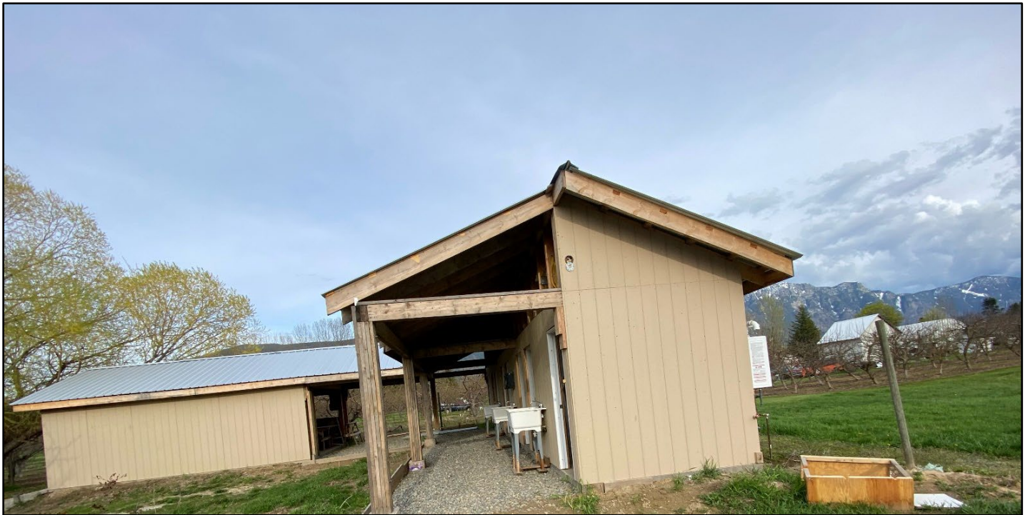
Figure 4: Photo of Existing Structure
