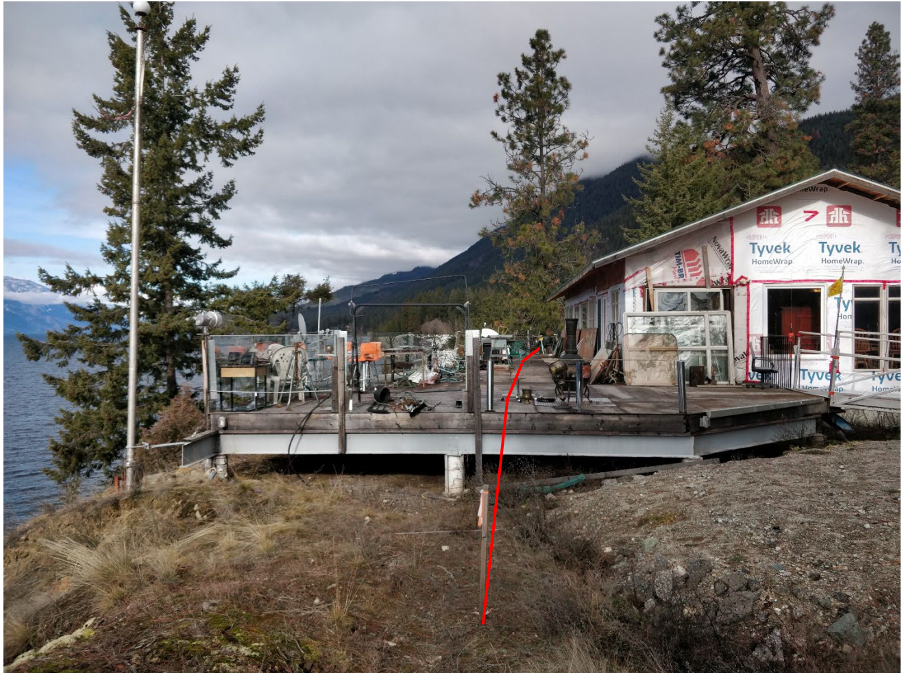
Figure 3 - View looking north towards the deck and dwelling. The red line shows the location of the 15 metre floodplain setback.
