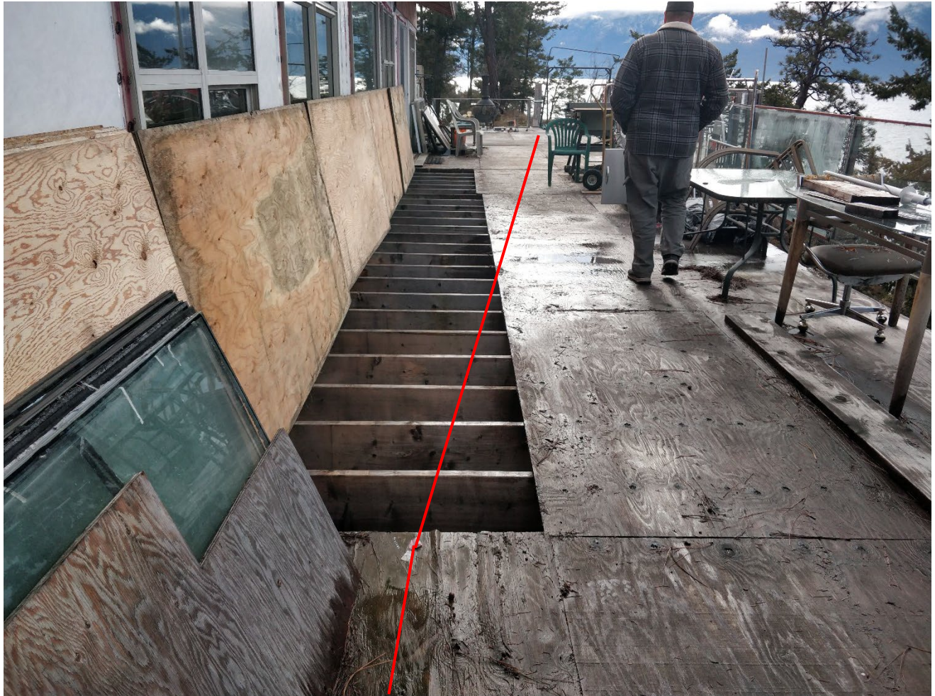
Figure 4 - View looking south from the deck. The red line shows the location of the 15 metre floodplain setback.
