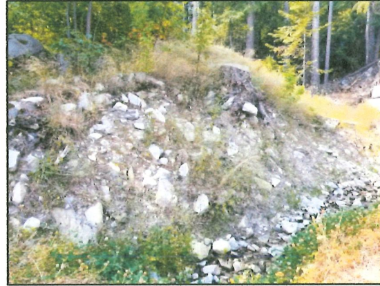
Photo 1. View of steep rocky slope on the west bank, Edwards Creek.
