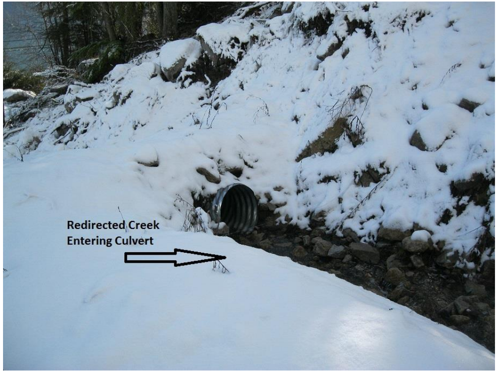
Figure 6: Edwards Creek directed through culvert
